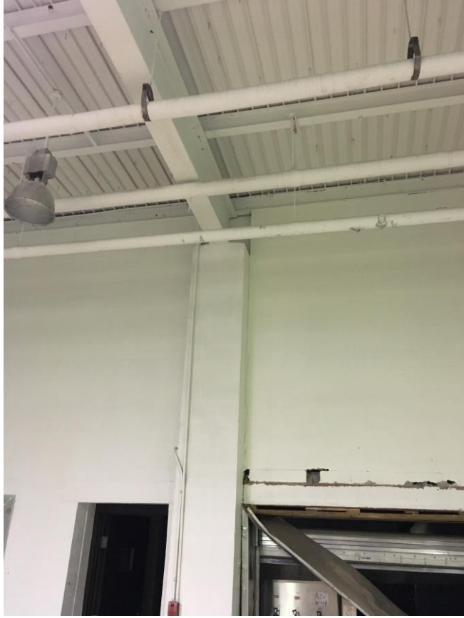
Picture 4: Steel beam supported roof
