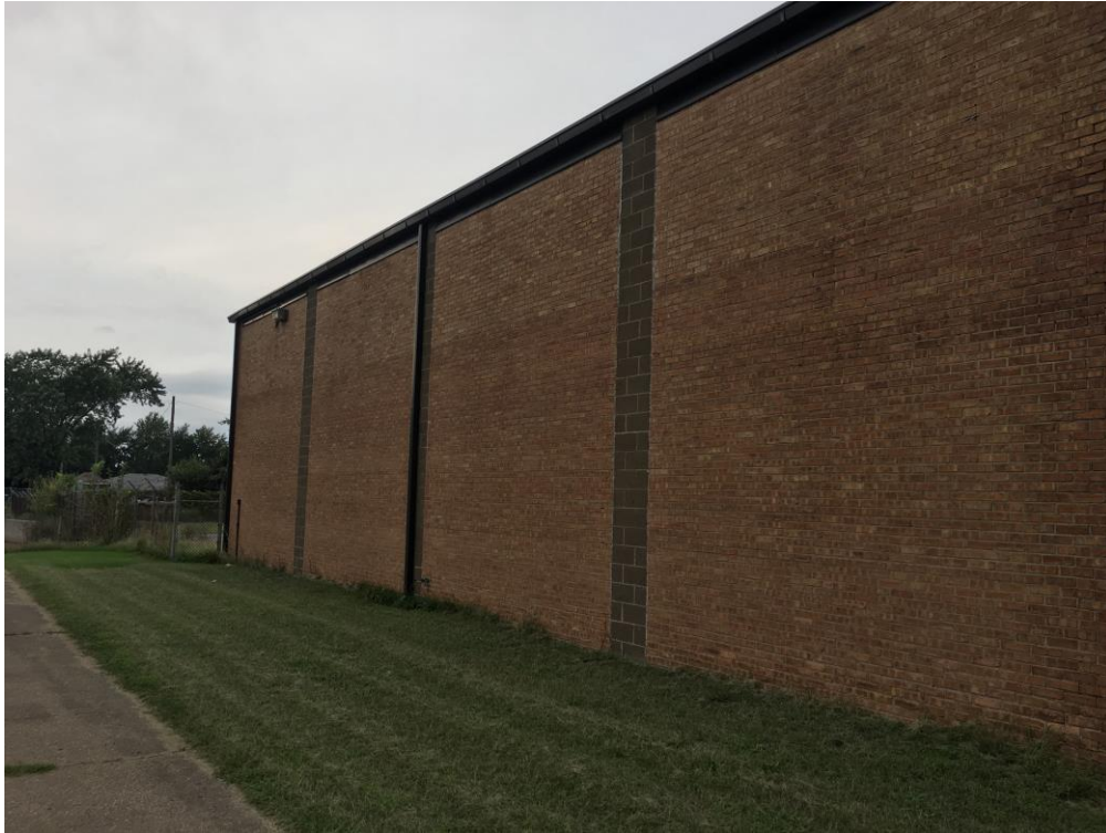
Picture 2: Masonry exterior walls and concrete interior walls
