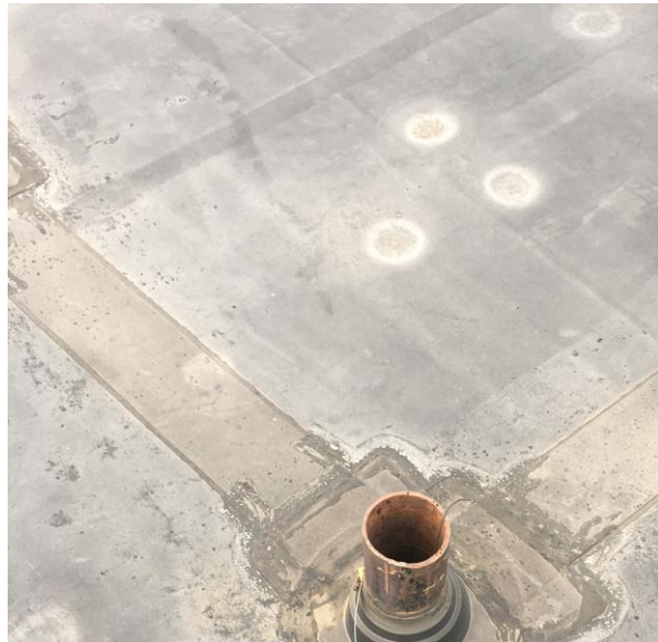
Picture 5 Asphalt Roof
