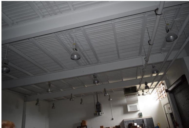
Picture 3: Steel beams in the gym
